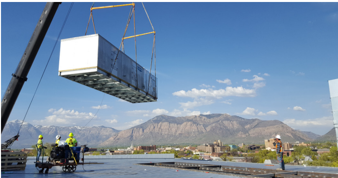
Installing Evapcold units is straightforward and reduces the amount of work performed by the refrigeration and electrical contractors.
