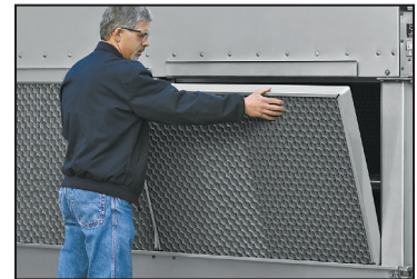
Framed Inlet Louver Design
