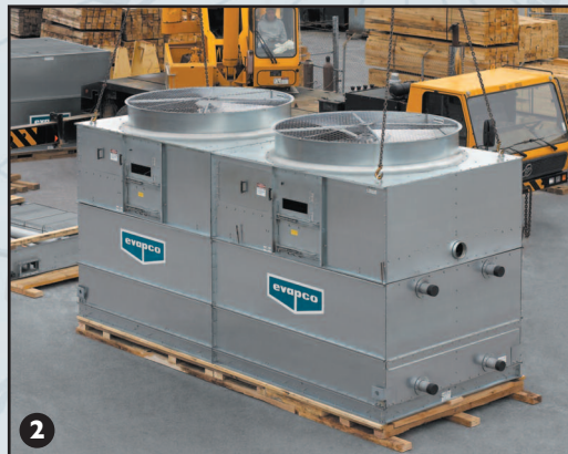
2 Mount Fan Section to Fill/Coil Section
