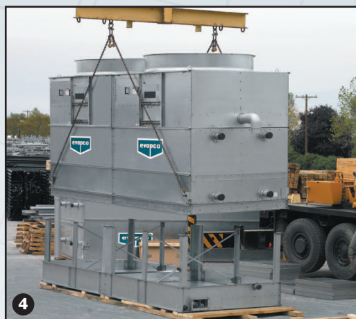
4 Mount Fill or Coil/Fan to Basin Section
