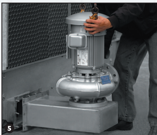
5 Mount Pump and Piping (Coolers and Condensers only)
