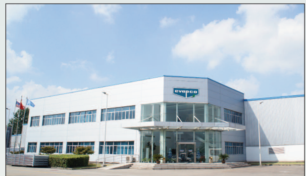
EVAPCO's Wholly-Owned Office & Factory in Shanghai, China
